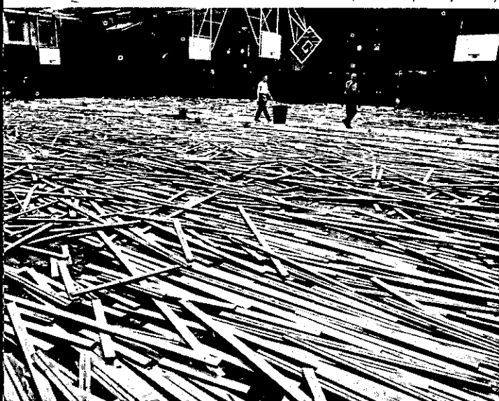
SCENE FROM THE PAST — This is the way the boys' gymnasium at Bethlehem Central High School looked in November, 1973, when all the floor boards had to be ripped up and re-laid or replaced. The severe damage was caused by the combination of a heavy rainfall and an electrical storm — loss of power meant the generator for the sump pump wasn't working, which allowed flooding water to seep into the gym interior. The bond issue now being proposed by the Board of Education includes money to pay for an auxiliary generator which would prevent re-occurrence of such building damage. (Photo courtesy of The Knickerbocker News-Union Star)
