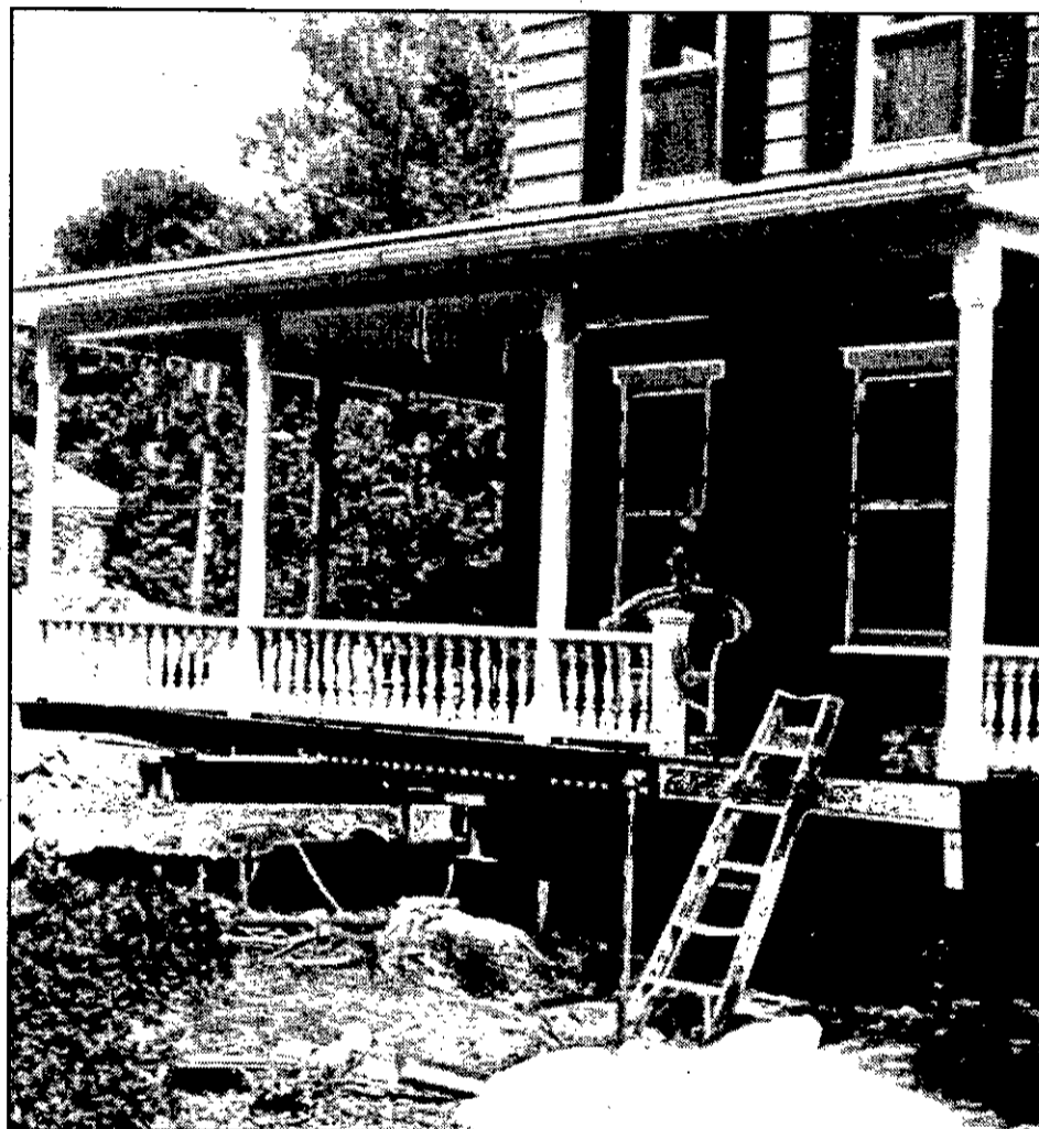
The Hoghe family's 112-year-old home at 346 Kenwood Ave. in Delmar stands on stilts as workers build a new basement and foundation underneath.
