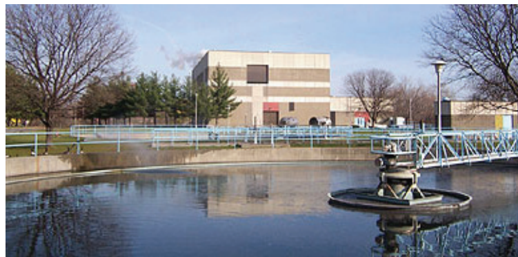
The North Treatment Plant in Menands.
