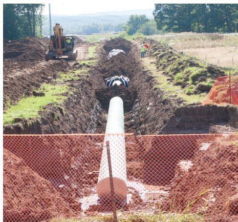
Contractors install new gas pipelines off of Meads Lane Thursday afternoon.
