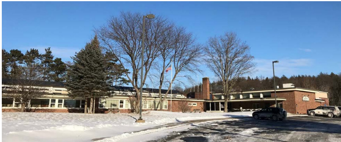
Assessed at $1.7 million by the Town of New Scotland in 2016, Clarksville was appraised at $410,000 in February 2017 and at $325,000 in January of this year.
