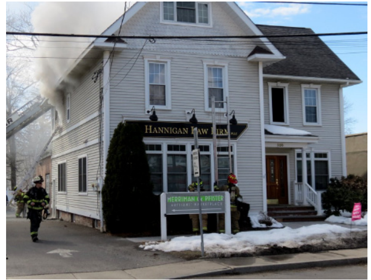
Crews battle a blaze at 388 Kenwood Ave.
