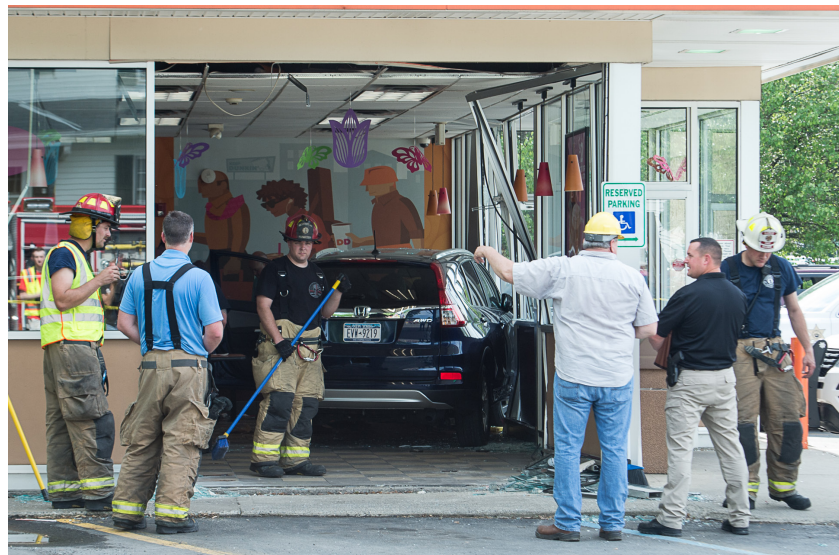
Cleanup continues after a vehicle drove through the side of the Dunkin' Donuts on Delaware Avenue Friday, June 1.
