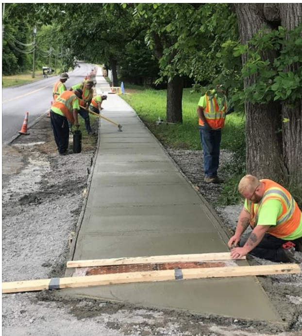
Town crews work on pouring a sidewalk.
