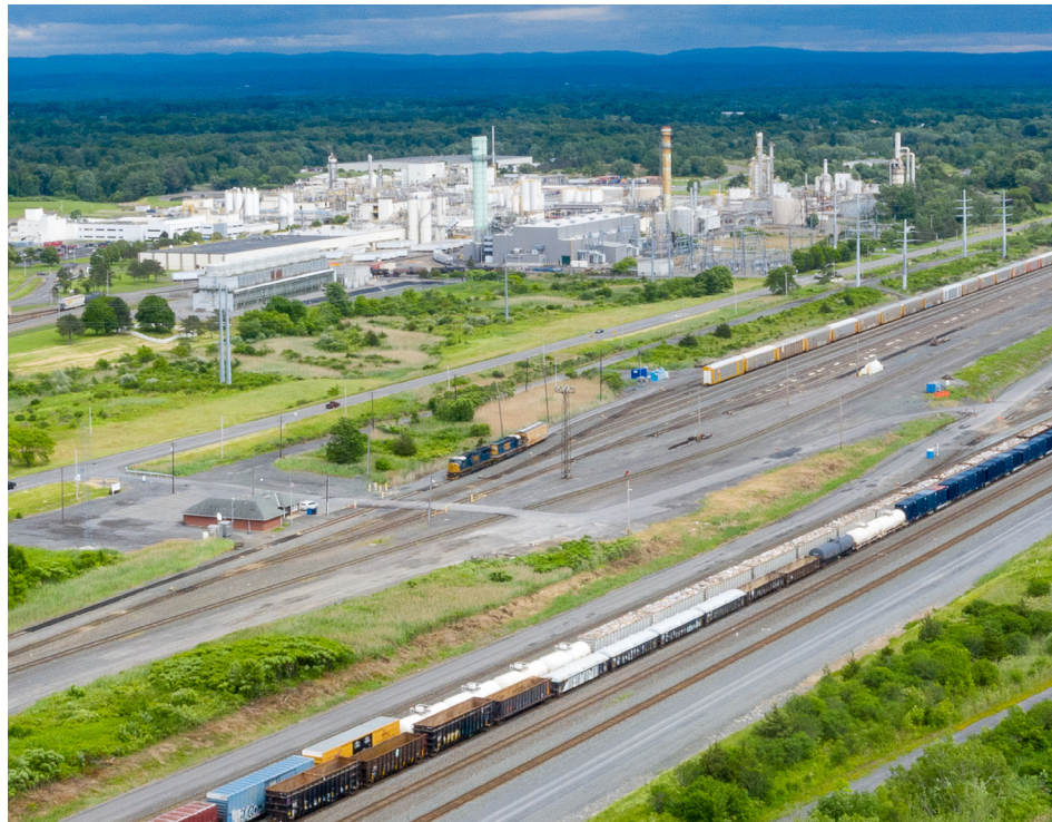
SABIC, Owens Corning and CSX make up a large portion of Bethlehem's industrial base in Selkirk. This arial photo is taken from the Feura Bush side of the CSX rail yard.
