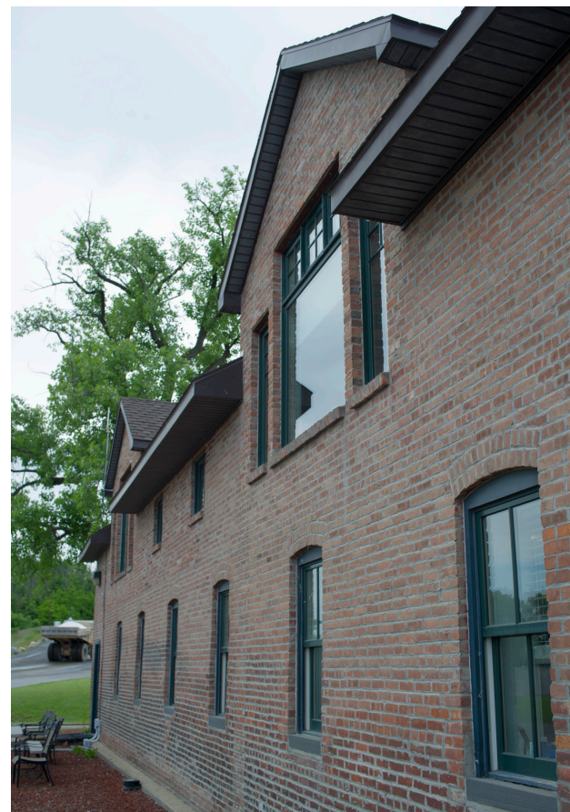
The old Sutton and Sutterly stables that the Port of Coeymans renovated now serves as the port's offices.
