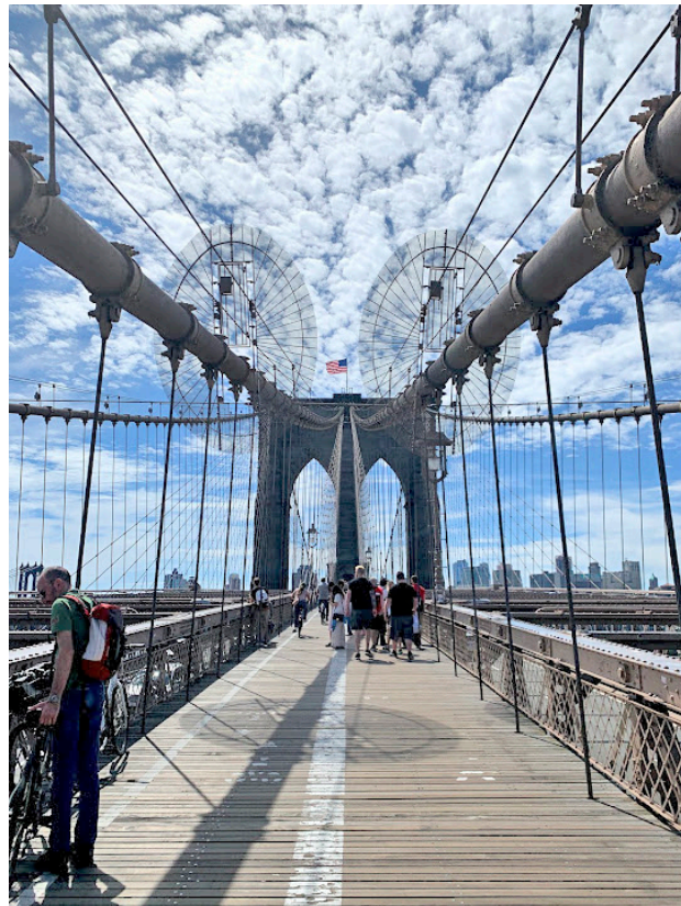
The Brooklyn Bridge, connecting Manhattan and Brooklyn over the East River, is one of many locations that people can access for free for scenic walks and photography opportunities. Diego Cagara / The Spot 518
