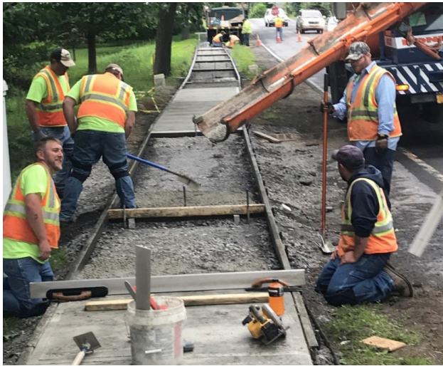
The town's Highway Department workers busy pouring a sidewalk. Submitted photo
