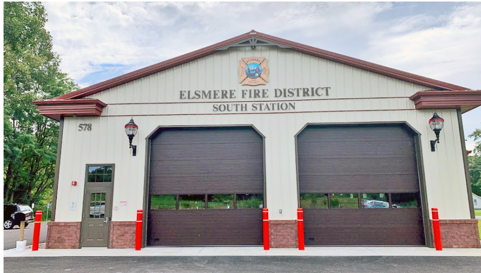
The Elsmere Fire District's new substation has technically been in service since Aug. 7 already.
