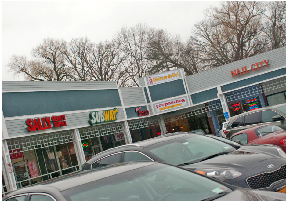
The stores at Delaware Plaza eagerly await holiday shoppers this week, but shopowners are now looking at how water line repairs will impact traffic. Diego Cagara / Spotlight News
