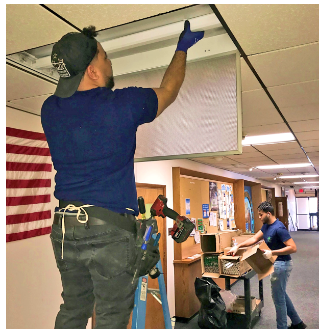
Bethlehem Town Hall switched to LED lighting last month.
