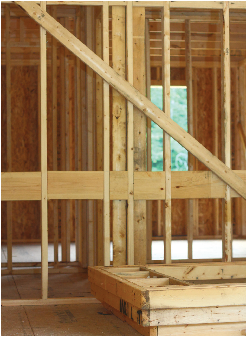
Many people now opt to stay in their homes and improve their properties rather than move out.
