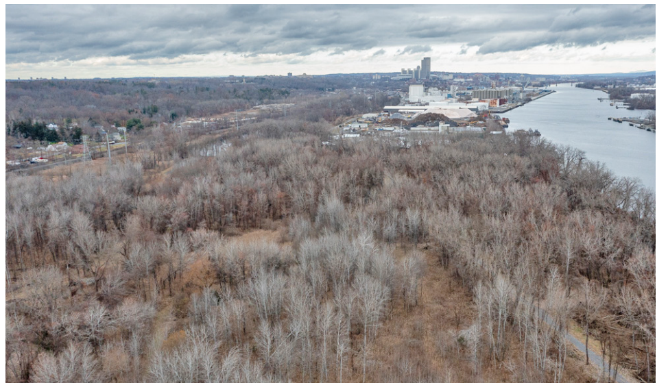
An aerial view of Beacon Island with the existing Port of Albany to the north. MarmenWelcon will be producing wind turbine towers here once the factory is built. Jim Franco/Spotlight News
