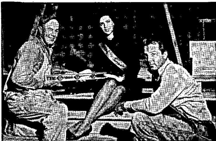
IT'S ON THE LEVEL — Construction workers J. R. Willig (L) and Douglas Bend (R) and Miss Colonie Center, Linda Cole, check to make sure the "Community Room" of the all new Colonie Center is really on the level. When completed the Community Room will accommodate 325 people and will be fully equipped with stage, sound system, projector, and screen. The Colonie Center Community Room will be available to local civic community organizations and clubs.
