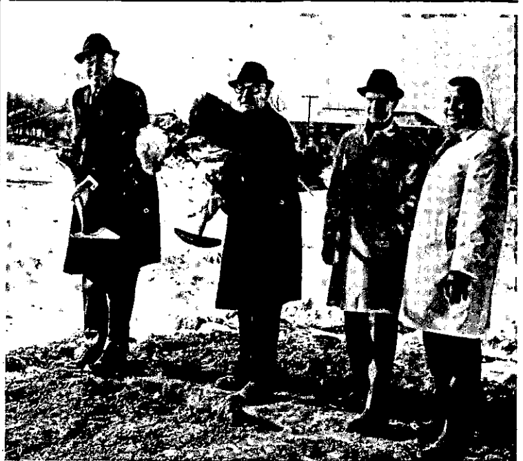
NOT SNOW! No, these men are not shoveling snow. They're breaking ground for the new $2 million Albany Dodge facility on a 9-acre plot on the south side of Central Avenue near the Everett Road Exit of the Northside Arterial. Left to right, Mayor Erastus Corning, R. Harold Craig, President of Albany Dodge; John D. Fulton, Executive Vice President, Greater Albany Chamber of Commerce; John Howell, District Manager for Dodge.
