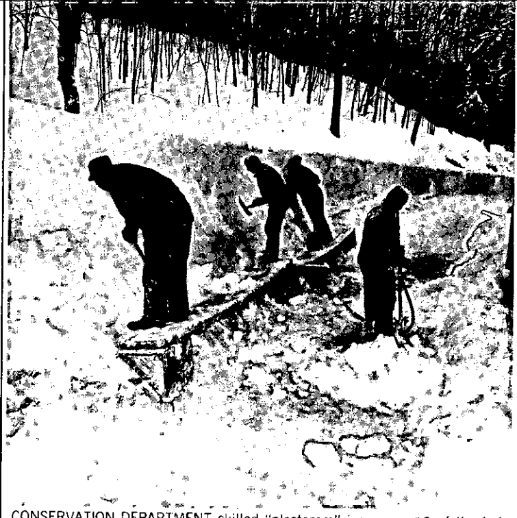
CONSERVATION DEPARTMENT skilled "plasterers" ice curve #6 of the bobsled run with slush as the worker in the center sights along the curve to check alignment.
