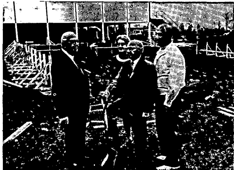
MEMBERS OF THE ALBANY JEWISH COMMUNITY CENTER will welcome the news that the promised outdoor pool has now reached the point of reality. Construction has begun on the new facility which will adjoin the present patio serving the indoor pool. The dimensions will be 45' wide by 75' long with a depth from 3 1/2' to 5 1/2' providing an extensive area for swimming. A diving area has not been included in this facility. There is a diving section in the indoor pool. In the photo above, Julius Muffson, Center President (leaning on shovel), hears Mr. Alexander, Building Committee Chairman, describe the progress of the new project. Standing next to Mr. Muffson is Betty Clark, Swim Director at the Albany Jewish Community Center, and at extreme right Al Stoman, Phys. Ed. Director.
