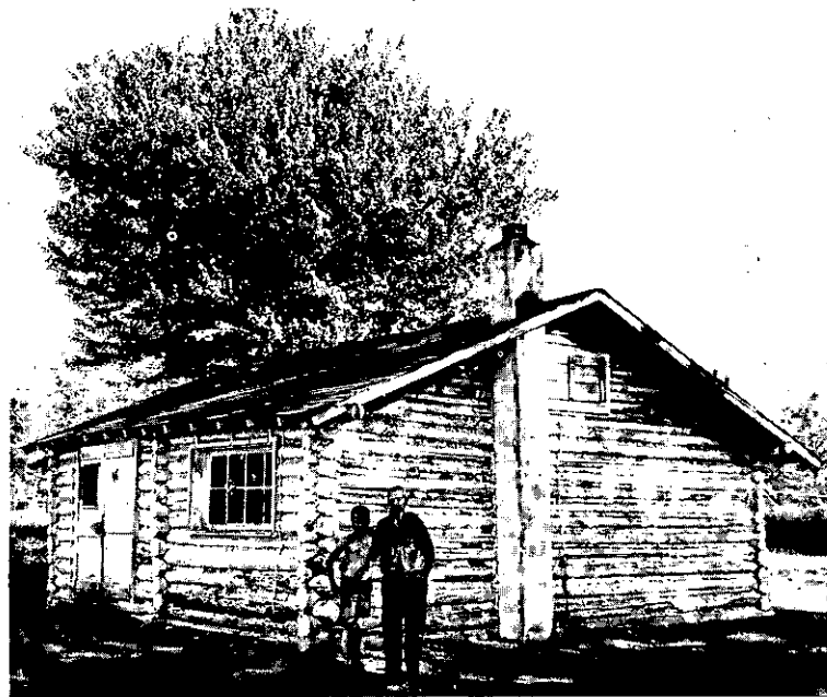
VOORHEESVILLE LAND MARK — Log cabin of retired R.R. worker Steve SITKOR was demolished to make room for new Voorheesville Shopping Center. Steve is pictured here with friend Billy Almy. The National Commercial Bank will be located in this spot.
