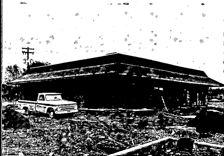
The nation's newest McDonald's at Delaware Avenue and Mason Avenue in Elsmere pictured under construction.
