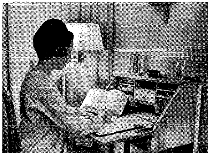
Floor model of BLBS study lamp permits student to place lamp out of the way, yet still have the light source in the correct position for illuminating work.
