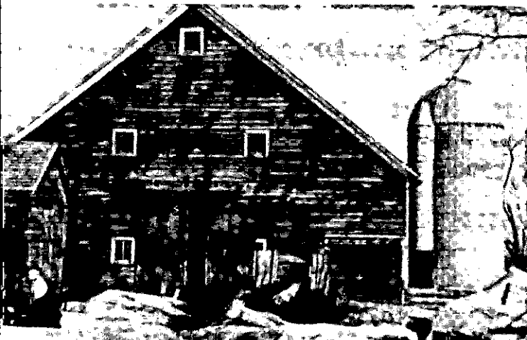
P. ZDIEBLOSKI BARN on Elm Avenue south of Rt. 32. A new roof was put on some years ago and the eaves were carried forward at that time.
