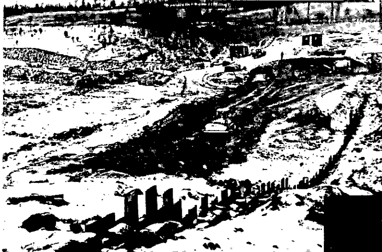
Beginning of the dam construction and scooping out of basin of reservoir.
