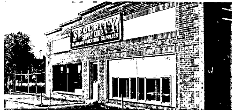
WHEN IT COMES TO plumbing and heating supplies, Selkirk again boasts one of the finest. Security Supply Corporation, with stores in both Albany and Schenectady Counties, is one of the larger area suppliers. The office and warehouse in Selkirk also supplies walk-in purchasers and enjoys a fine reputation both among area plumbers and businessmen and the many customers who have bought there over past years.
