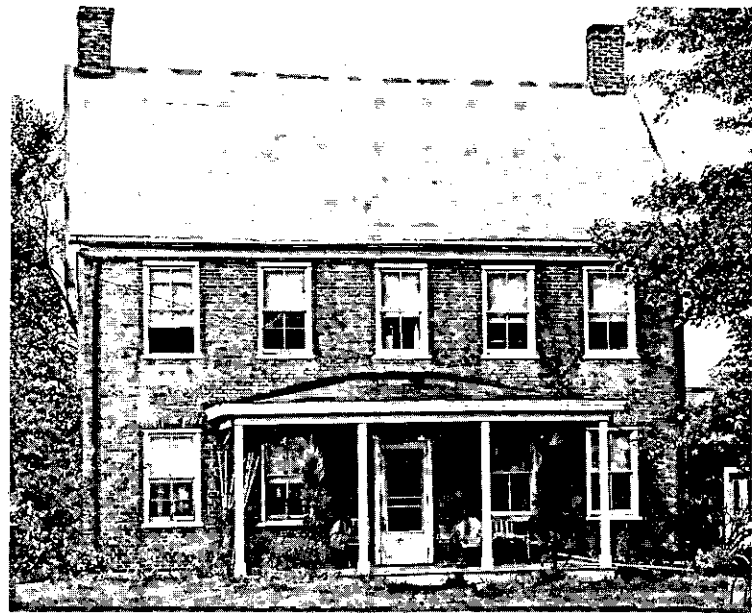
BECKER HOMESTEAD —this house was built in 1800 at Beckers Corners by Albertus Becker, grandson of the original settler, Albertus Becker, living along the "old" road from the Onesquethaw Creek to the Hudson River. Albertus W. Becker, grandson of the man who built this house, was Supervisor of the Town of Bethlehem in 1862.
