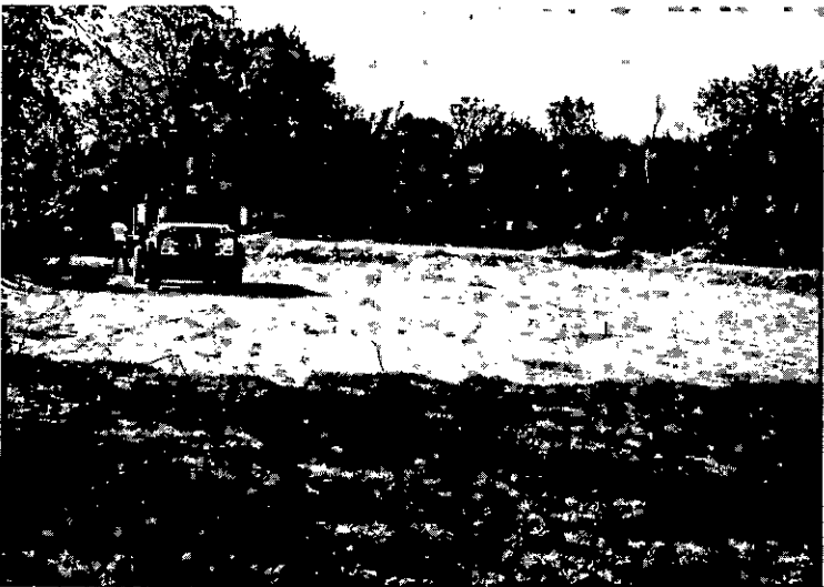
TOWN OF BETHLEHEM workers have cleared and leveled a space more than 100 x 60 back of the R-C-S Board of Education building in Selkirk. It will be blacktopped for basketball during the spring, summer and fall — and flooded for ice skating in winter. It's a sure bet that this new facility will not help to cut the amount of vandalism — in fact, the records show that these added facilities draw additional onlookers who, in turn, look for new things to destroy.
