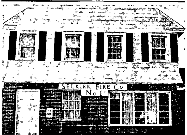
THERE'S A NEW SPARKLE to the Selkirk Fire Co. #1 fire house these days. It has all new aluminum siding and two new fire-proof doors, all installed by HRH Designs located on 9-W.
