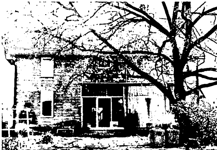
Slingerlands barn restoration project: keeping the character of a barn with living conveniences of a modern residence.
