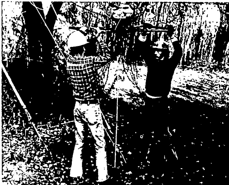
Bethlehem Video crew uses motor-driven winch to drive anchor.
