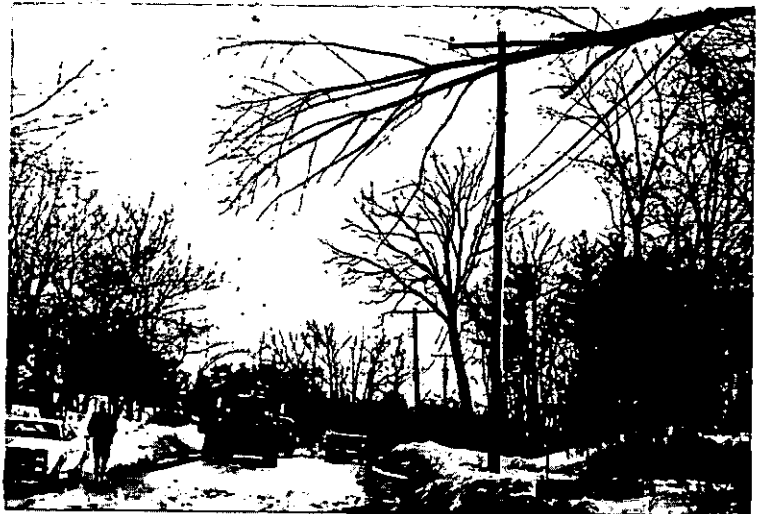
Wind-blown tree limb cuts power on Feura Bush Rd.
