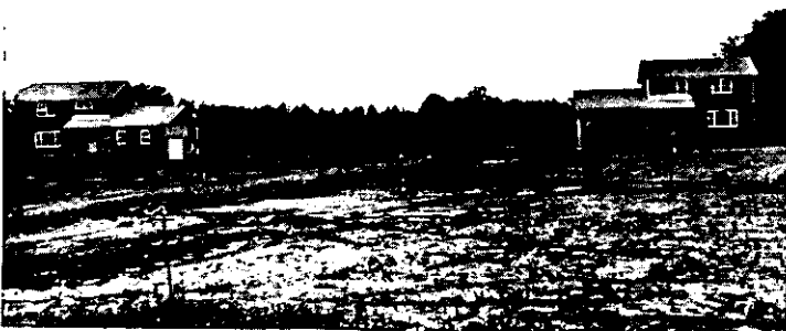
Homebuilding in Delmar: the first two of 131 single-family dwellings planned for the Brookfield subdivision behind Brockley Dr.
