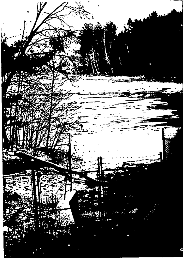
Part of the Bethlehem reservoir, currently at a 12-year low, but catching runoffs from the Helderbergs (culvert in foreground).
