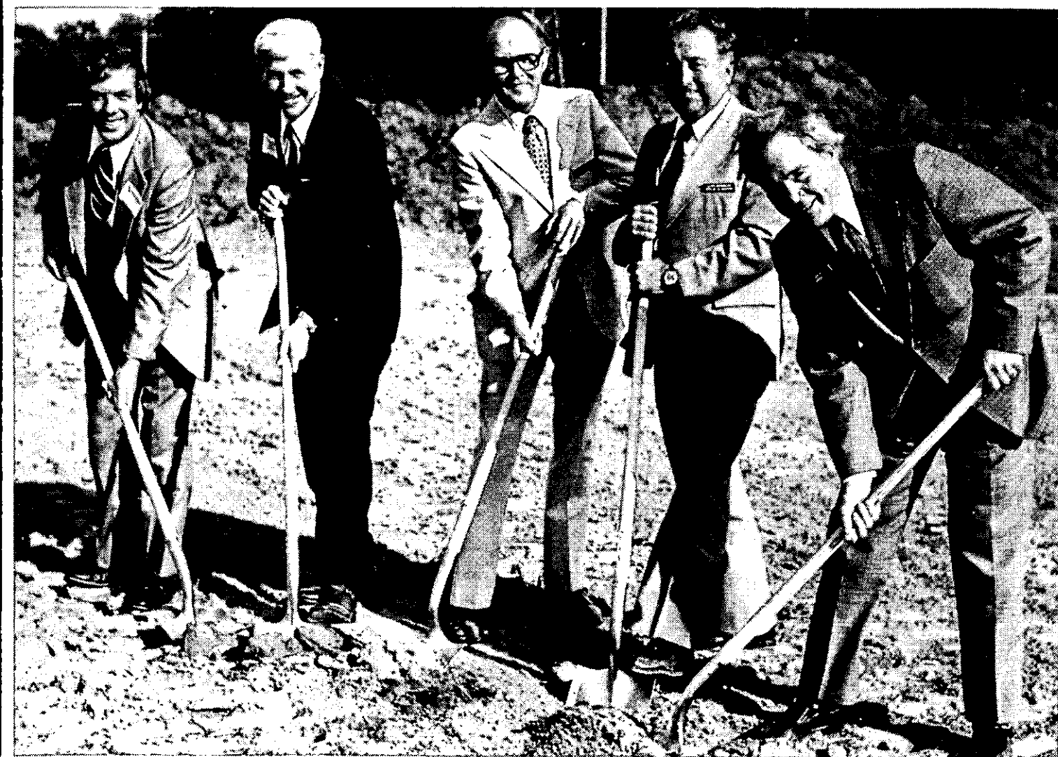
Groundbreaking in Glenmont
