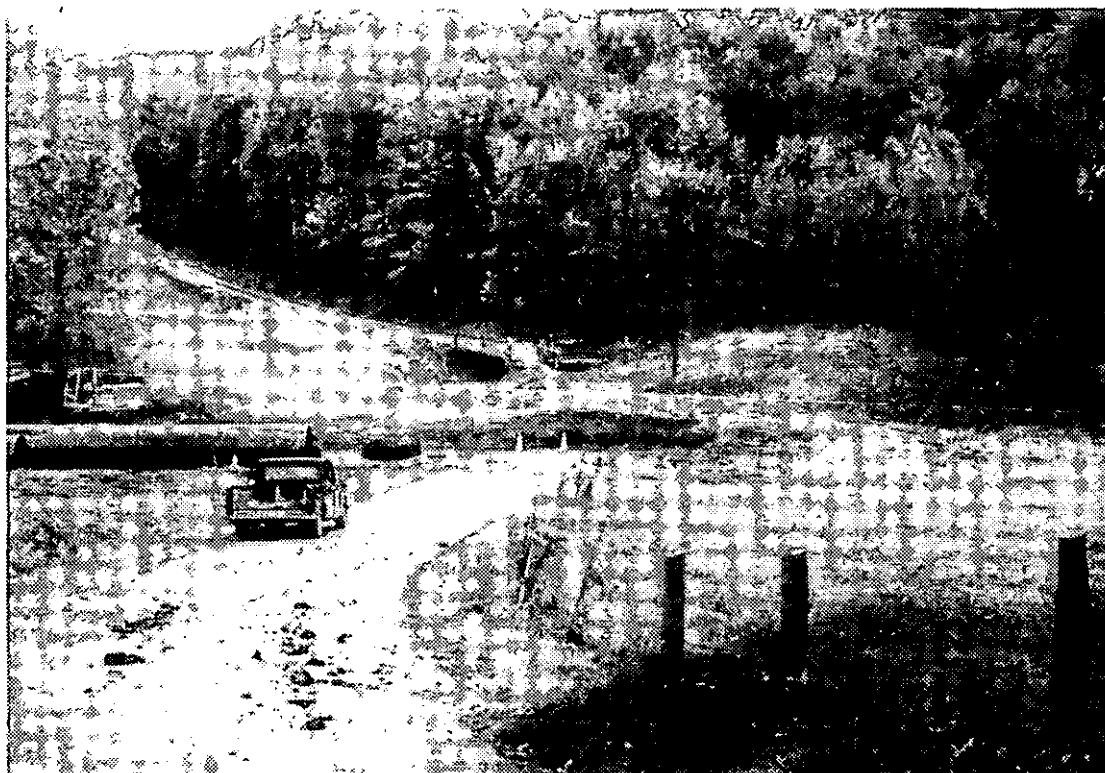
Bethlehem highway workers last week laid the first of three large pipes to carry the Philippinkill under the relocation of VanDyke Rd. in Delmar. The rusted old bridge, center, the only bridge maintained by the town, will be removed. (More photos on next page).
