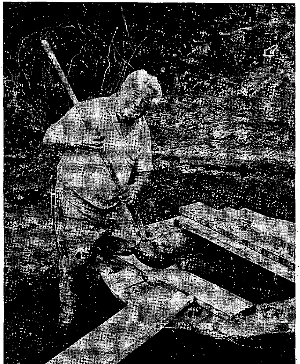
Tony Mauro finishes up work on the town's deepest manhole.
