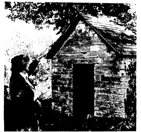
Original door is intact in the stone smoke house near the farmhouse.
