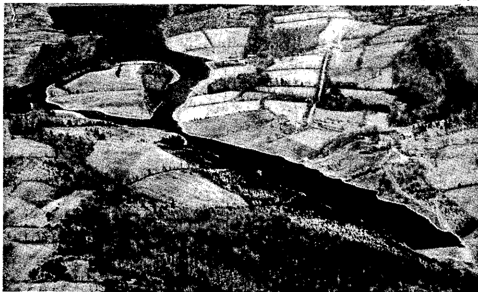
Bethlehem's Vly Creek Reservoir. The proposed natural gas pipeline would go through the southern leg of the reservoir, on the lower right in this picture.
