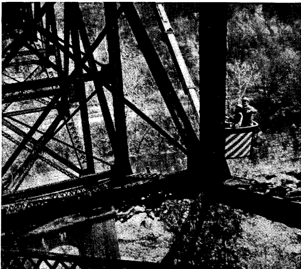
Bill Hadersbeck, left, a bridge inspector for the state Dept. of Transportation, and Dave Cox, bridge engineer, use a "cherry picker" to show media reporters and photographers why the Rt. 9W span over the Normanskill has been posted for vehicles over five tons.
