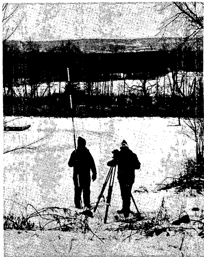
Engineers and surveyors for the Tennessee Gas Transmission Co. were in New Scotland last week plotting the route proposed for the new 30-inch line that will parallel the 24-inch line that was laid across Bethlehem and New Scotland in 1951. Above, Henry Dinelle of Ludlow, Mass., left, works with Nick DeCesare of Agawam, Mass. on the transit just off Clipp Rd. On the cover: A Tennessee Gas helicopter last week carried the project's chief engineer on an aerial survey of routes that by-pass the Vly Creek reservoir avoiding private wells and springs.
