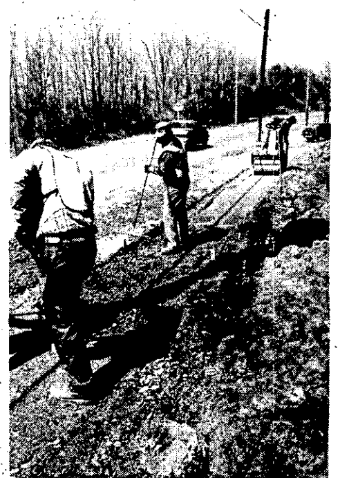
Town workers prepare a section of the new sidewalk on Elm Ave., installed to eliminate hazardous walking conditions for students on their way to the high school.
