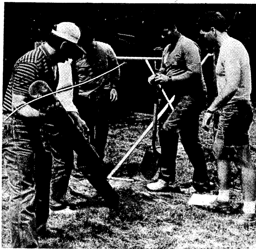
Volunteer parents were installing a new fitness trail at the Glenmont School Saturday, hampered somewhat by subsurface water in the field behind the school. Among those working in the hand walk station are Dan Fero and Sepi Constantino, supervised by phys ed teacher John Furey. The equipment was donated by parents, teachers and Farm Family and Travelers insurance companies. Spotlight
