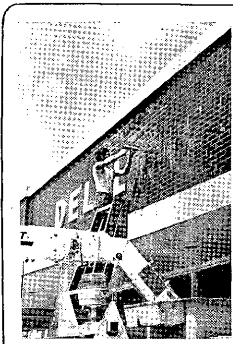
Meanwhile, the changes on Delaware Ave. continue. At left, a workman puts a new sign on the Del Lanes building after the bowling alley removed its old roof sign to get a jump on one of the recommendations of the Delaware Ave. task force. Delaware Plaza is also planning to take down its large
