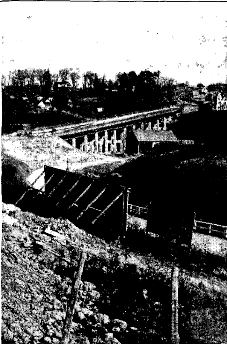
The present bridge carrying Delaware Ave. over the Normanskill was built in 1928, superceding the concrete structure that is still in use immediately below the Delaware Ave. bridge. That bridge, built in 1911-12, replaced an iron bridge erected by the town after the turnpike company gave up the toll road. Note the absence of heavy construction equipment in 1928.
