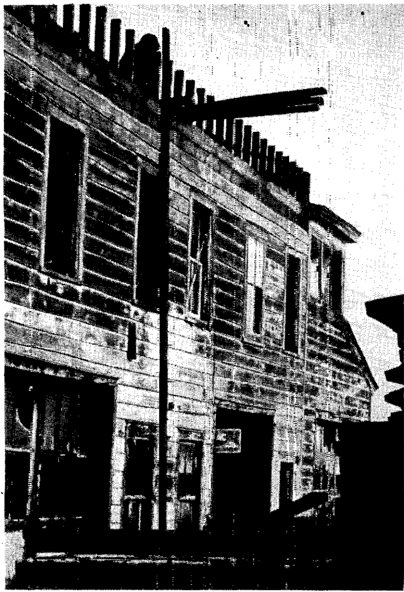
A Feura Bush landmark came down, piece by piece, last week, as Rothauit Garage, once an early Ford dealership, was disassembled to make way for a new post office. Owner John Flach, of Flach's Power Piping in Glenmont, said the new building should be under construction in March. Other stores may be added to the building, he said
