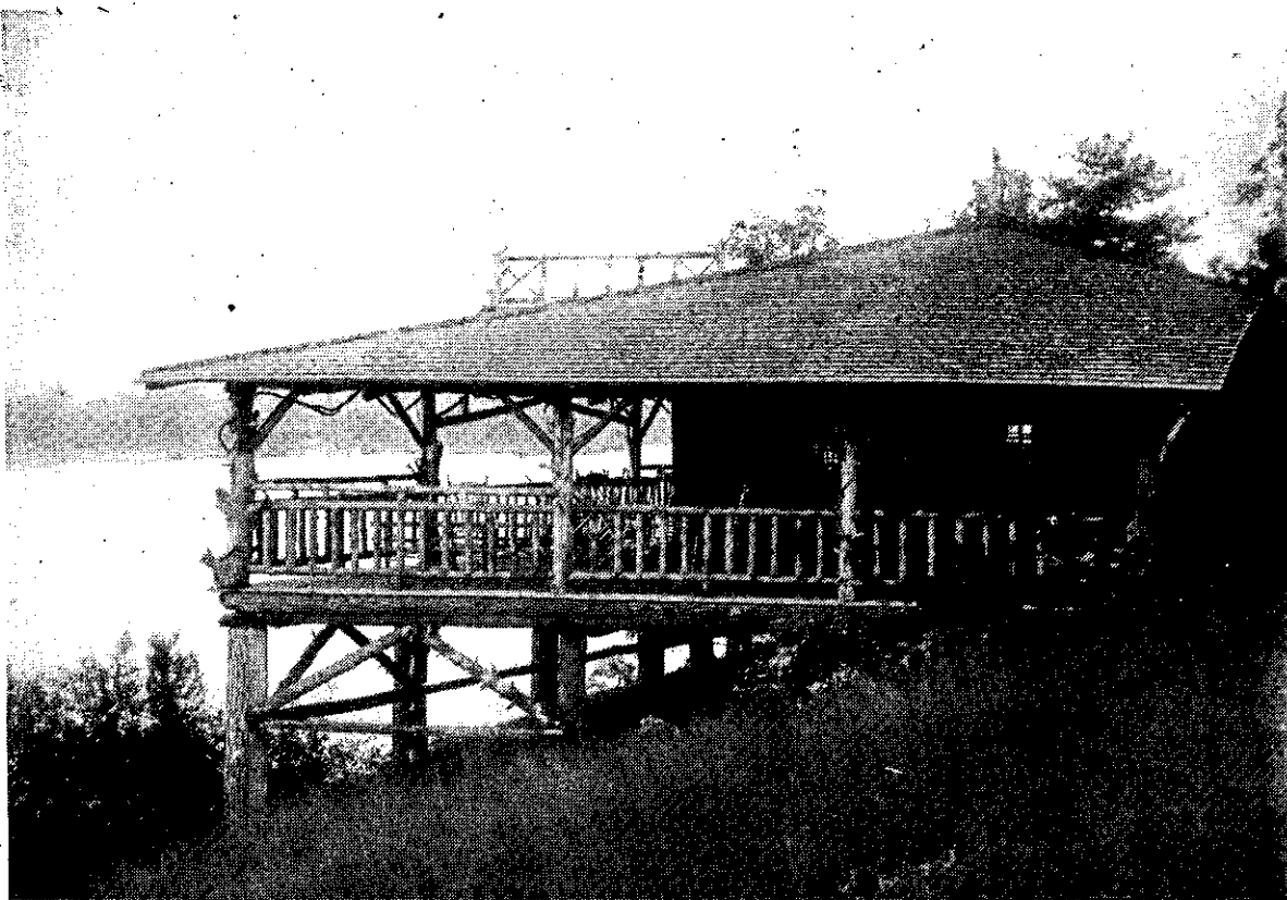
The rustic bungalow on the Lyons Estate, overlooking the Hudson River.
