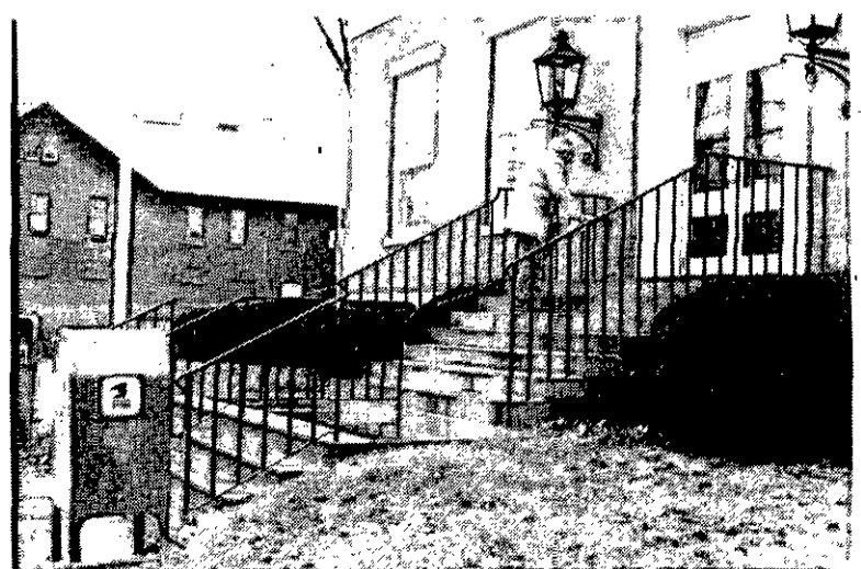
The front lobby of the Delmar Post Office is off limits to many disabled people in the community.
