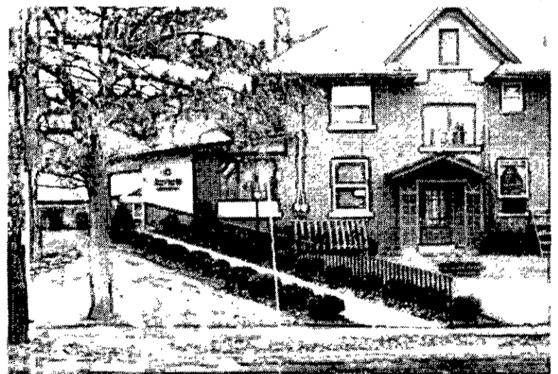
Drs. Marvin and Greg Sagor recently installed this handsomely landscaped ramp for handicapped access to their office at 50 Adams Place.
