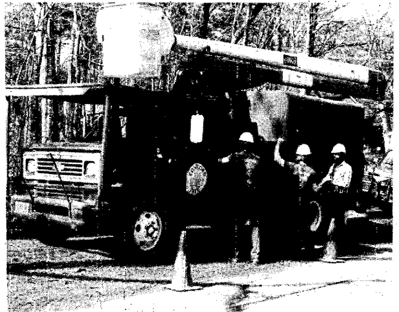
Lee and two workers first make the work site safe by setting out traffic cones around the service trucks set beneath the tree. Before acquisition of the bucket truck which reduces this two-hour job to a 30-minute one, Lee's men would free-climb the tree with the use of climb lines but not spurs that would damage the live tree.
