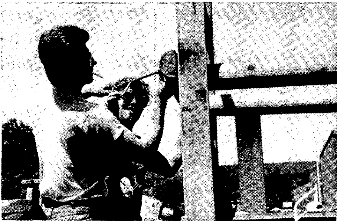
Jim McCooey, left, and Bob Griffen of the Clarksville Elementary School's PTA lend helping hands to the school's playground raising on Saturday at the school. The construction of the $8,800 wooden playground is the final step of 13 months of planning. At 6:30 p.m. on Thursday, the
