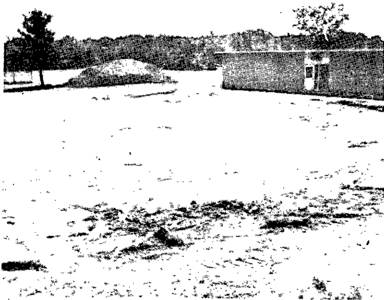
Excavation and site work has begun at the north side of the Glenmont Elementary School in anticipation of the relocatable classrooms. First graders at the school are expected to start using the classrooms during the third week of September.
